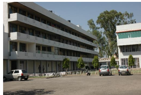
Three Storeyed Hostel Block
